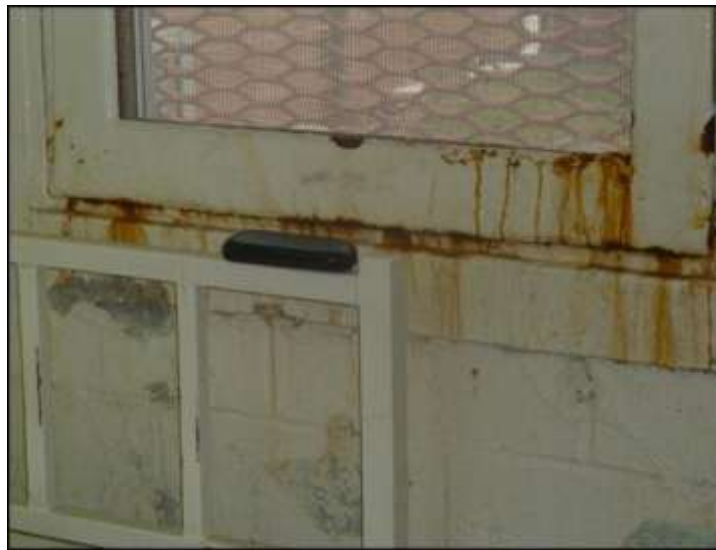
Window frame in a cottage cell
