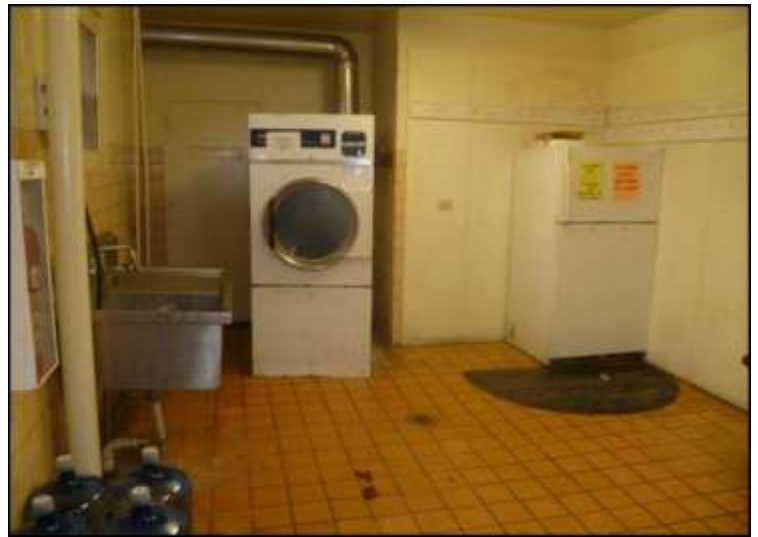
Cottage dryer and refrigerator
