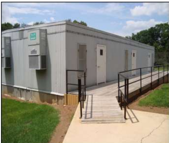
Outside school building
