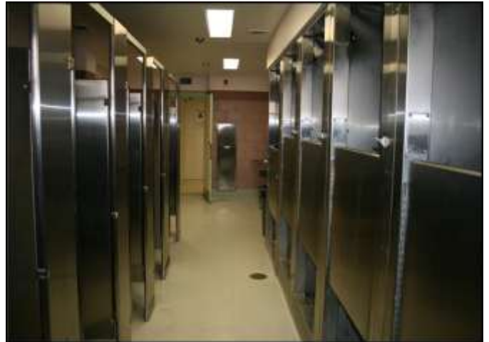
Renovated bathrooms on the A-Wing secure program
