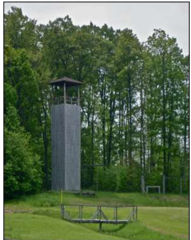
Outdoor recreation area and climbing tower
