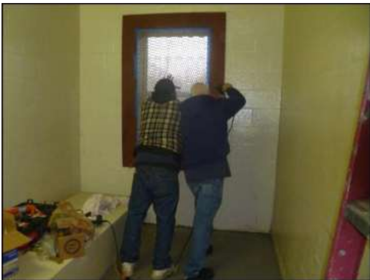
Window frame replacement is underway
