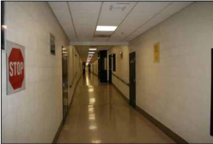
Hallway connecting three housing pods
