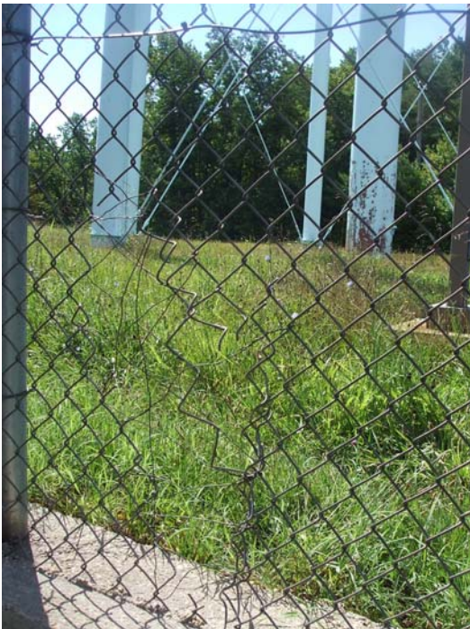
Hole cut into fence during for the escape
