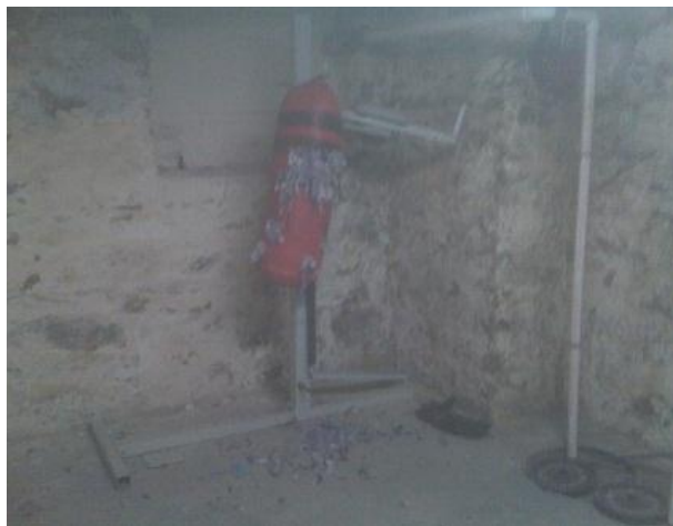
BASEMENT BEFORE RENOVATION
